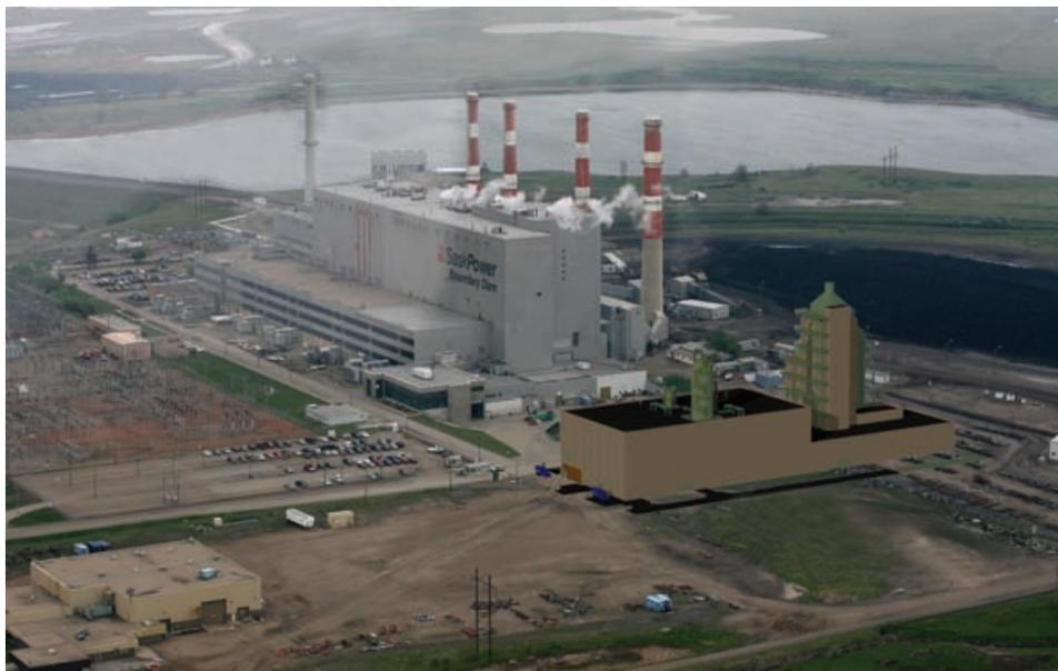
Figure 1: CAD Overlay of Future Carbon Capture Plant
